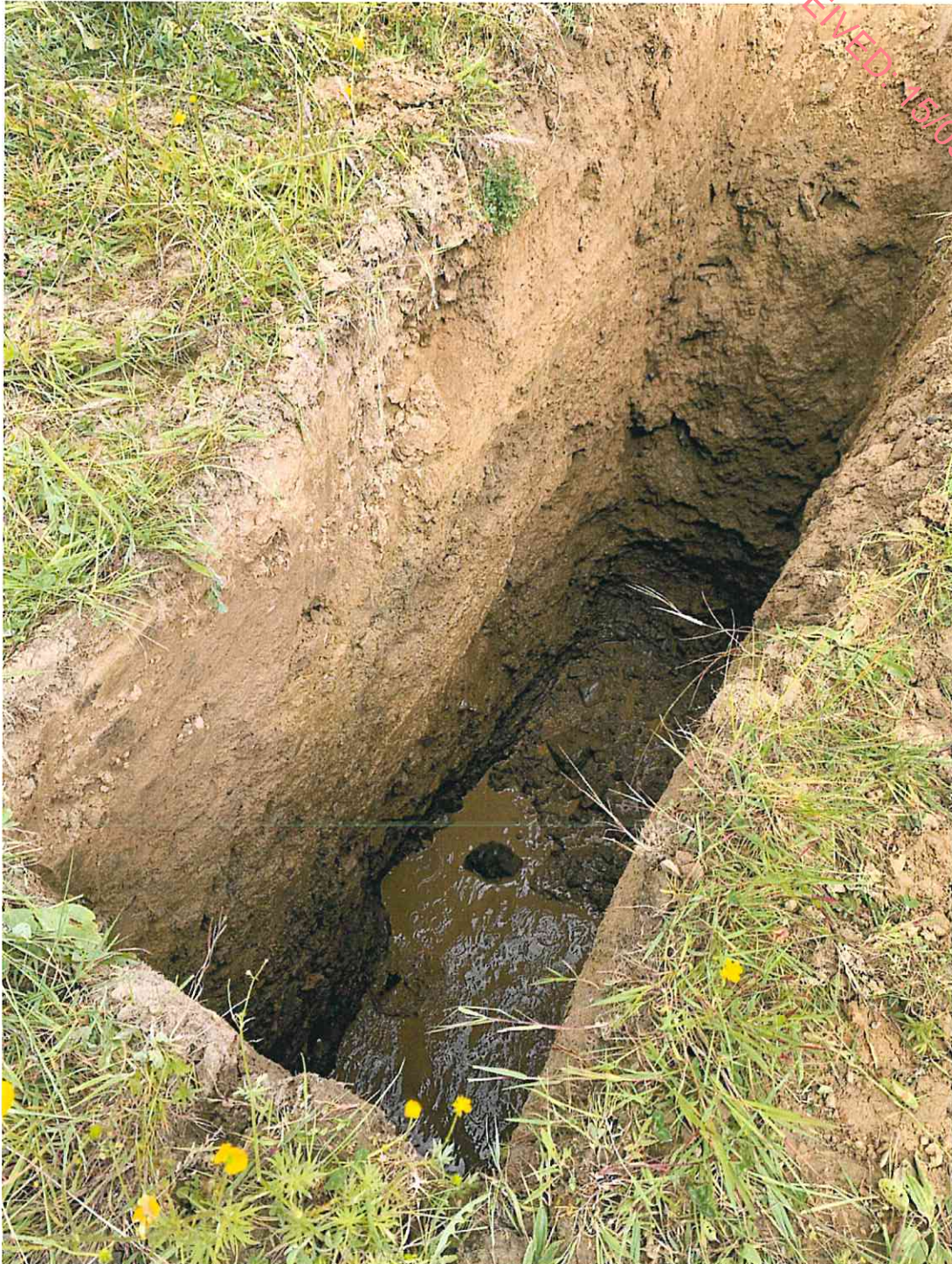
Picture taken after soakaway.
