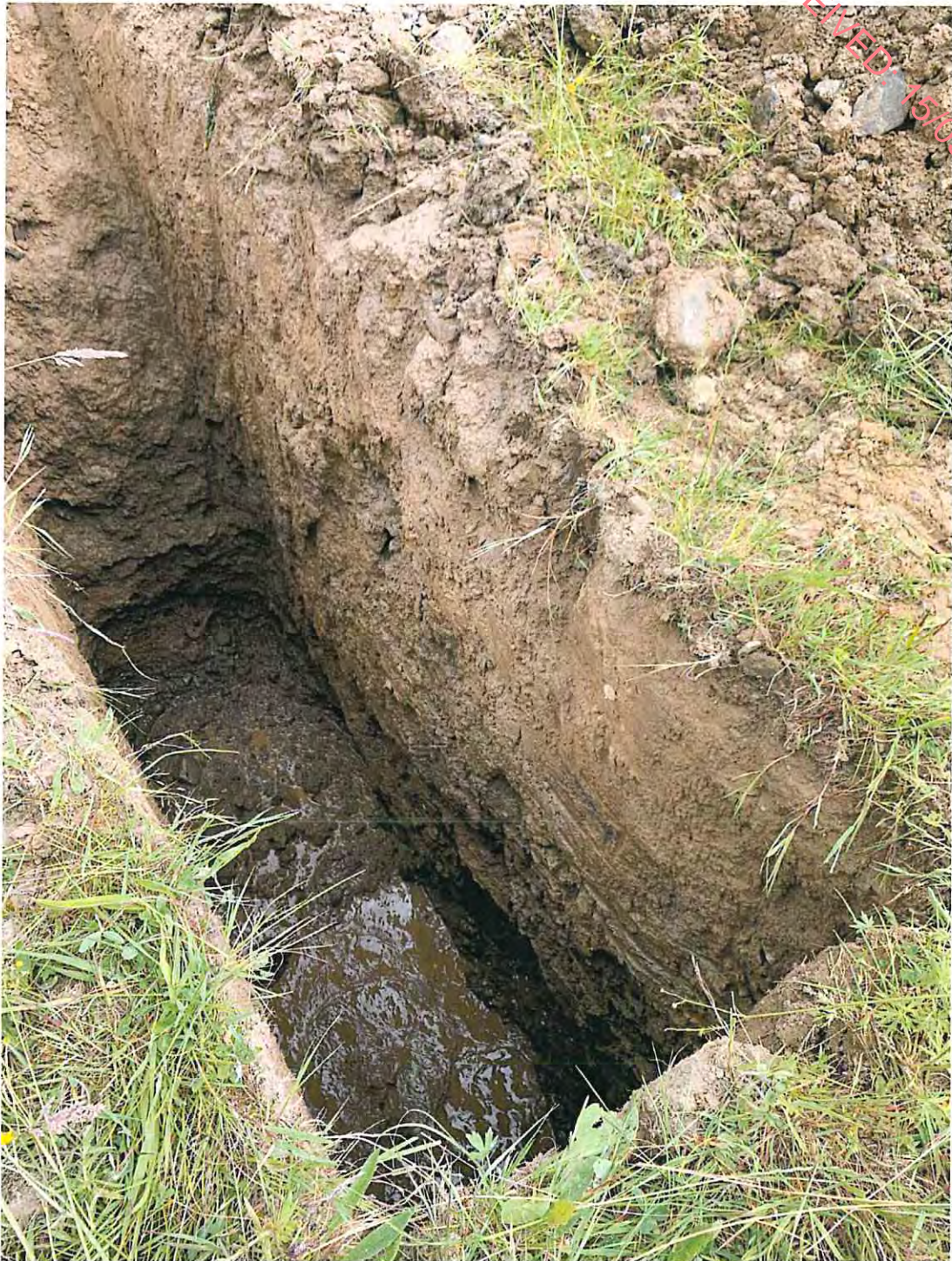
Picture taken after soakaway.
